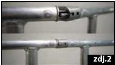
zdj.2 Closing base lock Fig. 2
