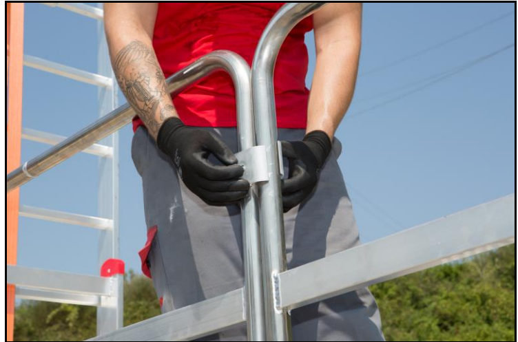
Fig.7: Installation of railings between two consecutive railings
