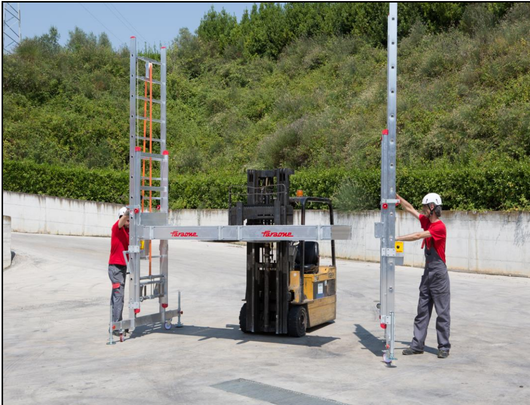
Fig.3: Inserting the deck between the two sides
